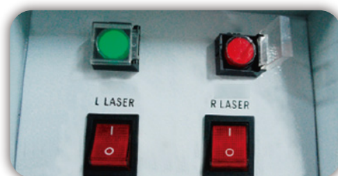
Image 2 - Manual control panel
